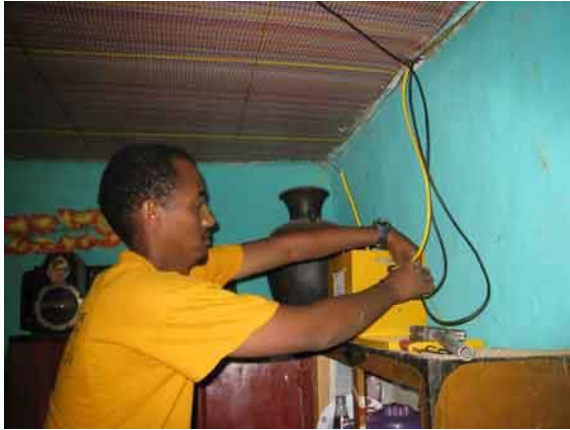
Installations in Ethiopia
