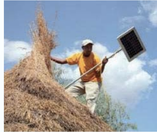
Installations in Ethiopia
