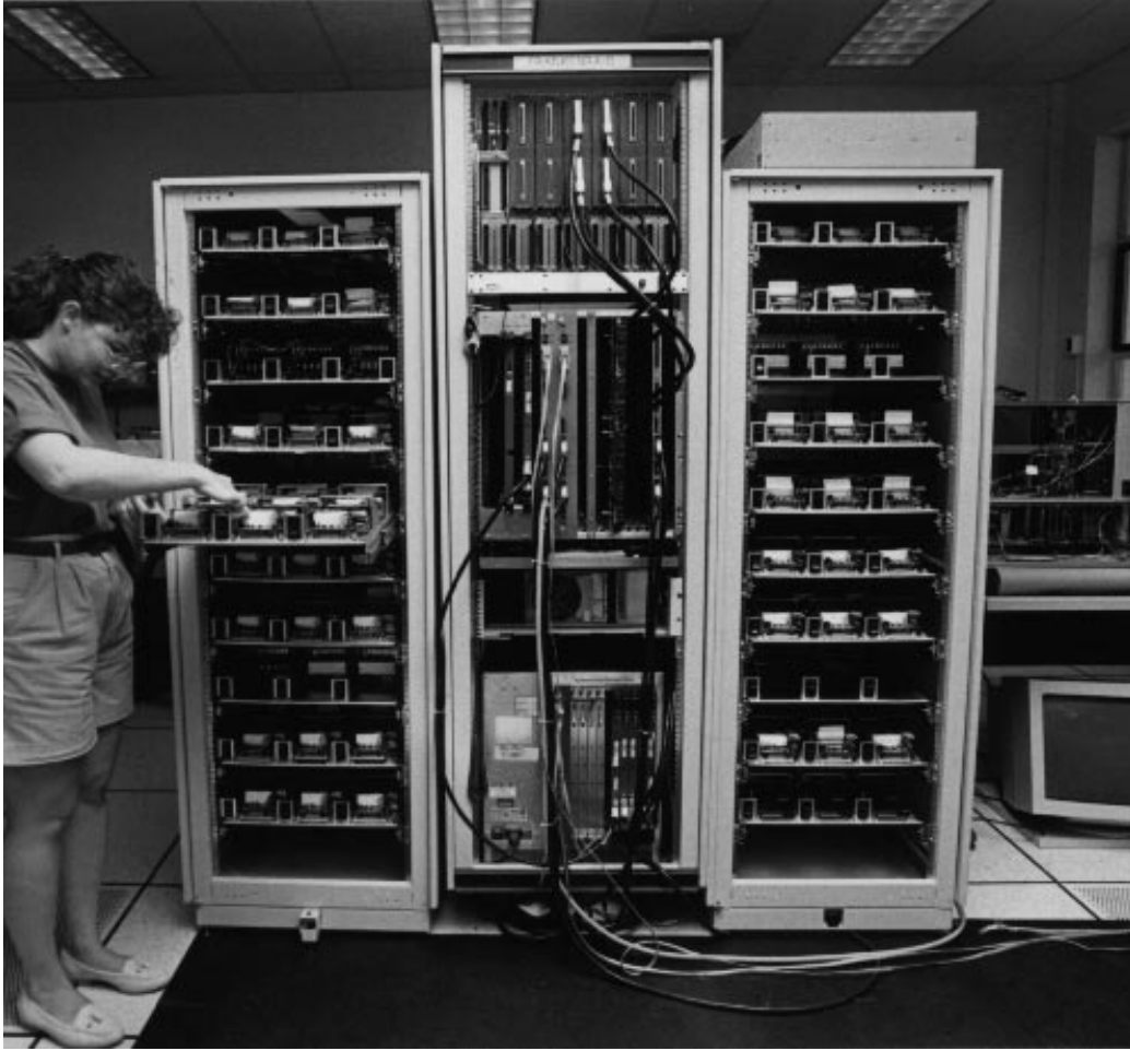
Figure 3: The physical packaging of the RAID-II File Server. Two outer racks contain 144 disks and their power supplies. The center rack contains three chassis: the top chassis holds VME disk controller boards; the center chassis contains XBUS controller boards and HIPPI interface boards, and the bottom VME chassis contains the Sun4/280 workstation.
